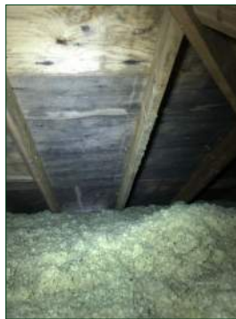
Microbial Growth on Roof Sheathing
