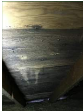
Microbial Growth on Roof Sheathing
